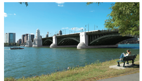
Longfellow Bridge, Boston, MA
