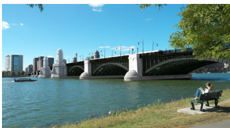
Longfellow Bridge, Boston, MA
